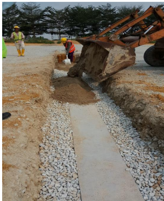
Fig. 5. Use of chipping to replace sand layer
