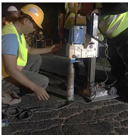
Fig. 7. The asphalt layer needs to be cored first before inserting the injection pipe into the ground.
