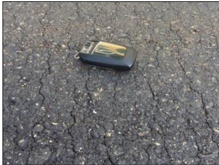
Fig. 1. Fine cracks formed on asphalt pavement due to the compaction at low temperature.
