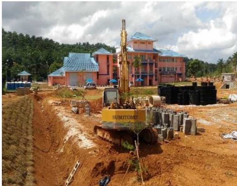
Fig. 6. Excavator during swale construction at PULAPAS
