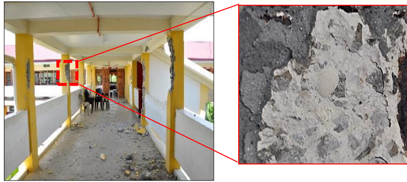
Fig. 1. Spalling and delamination at the 2nd Floor columns. Seashell was observed in the concrete.
