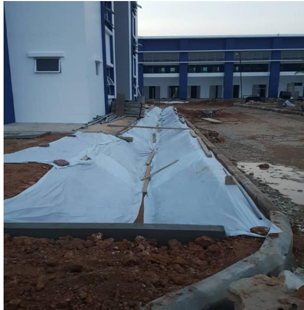
Fig. 8. Protective plastic covering during grass planting at IPD Pasir Mas
