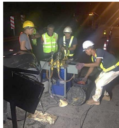
Fig. 8. Injecting the PU foam by mixing the two-liquid resin in situ into the ground.
