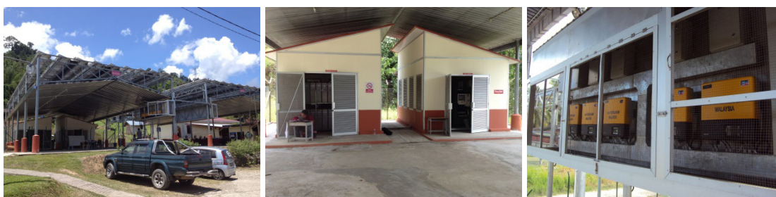
Fig. 3. SPVHS for rural schools in Sabah with a capacity of 40.32 kWp at SK Matupang, Ranau (left); a system's power house at SK Tg Paras, Lahad Datu (centre); and a grid inverter system at SK Sungai-Sungai, Beluran (right).
