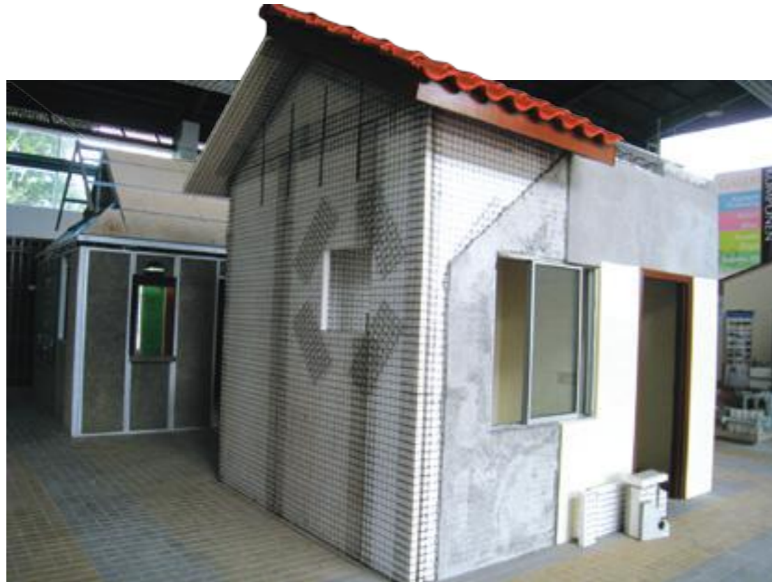
▲ A small house made with prefabricated walls is one of the exhibits at CIDB's IBS Component Gallery. This as well as other exhibits are used to train IBS students.
