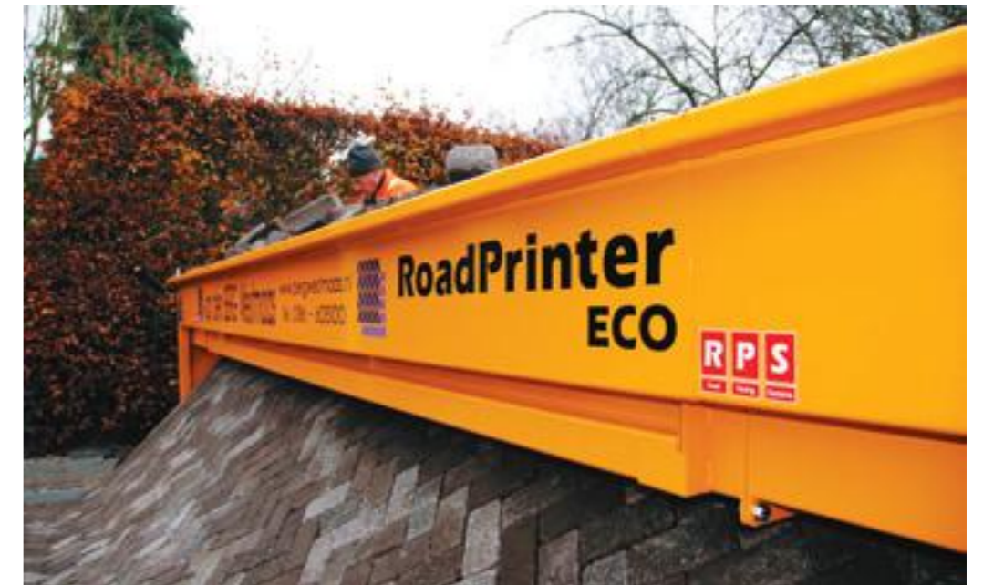
The RoadPrinter is set to revolutionize the way brick walkways and roads are constructed.
