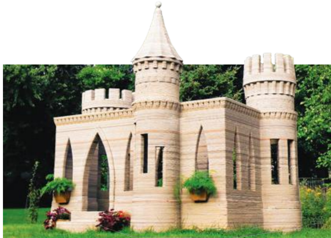
▲ 3D printing is the latest technology utilised in IBS. Andrey Rudenko of Minnesota in the United States for instance has managed to build a castle measuring 15 square metres using this technology and aims to 'print' a full-live-scale home in the near future.
