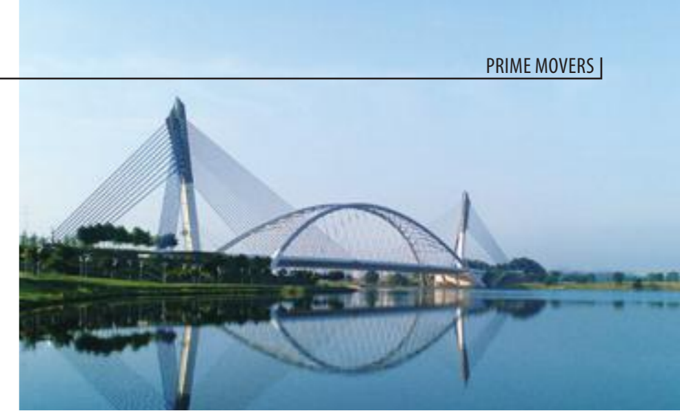
While adoption is slow, the Malaysian construction industry has already recognised the benefits of IBS, and developers and contractors have implemented a number of projects using IBS, such as the Putrajaya Bridge (pictured), Petronas Twin Towers and KL Sentral.
