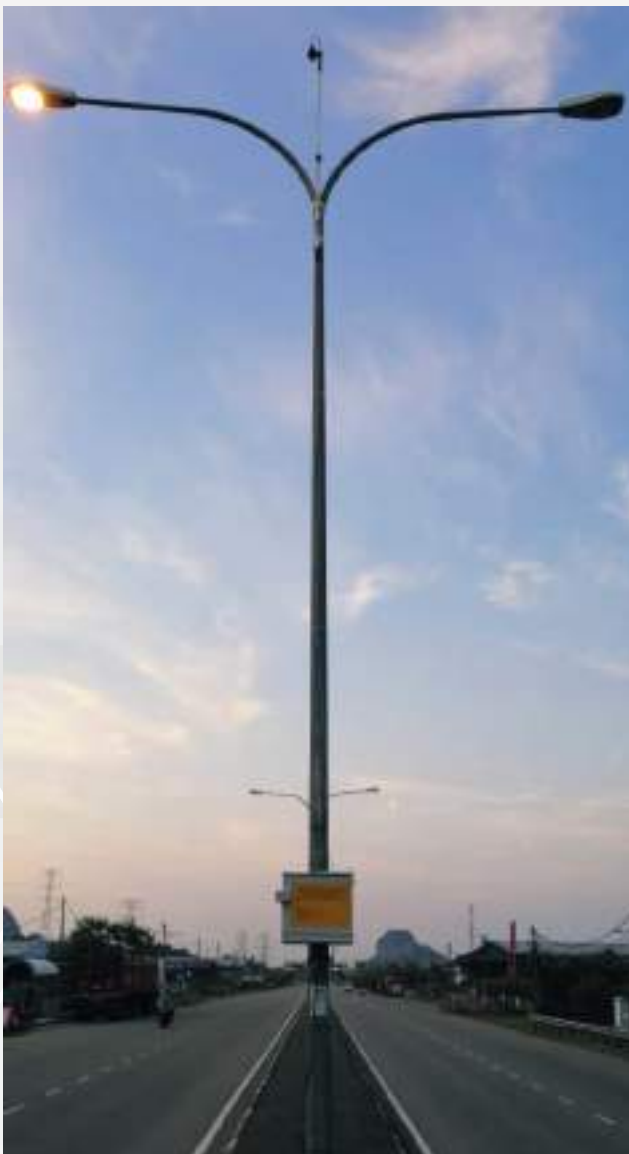
Figure 4: Installation at site
