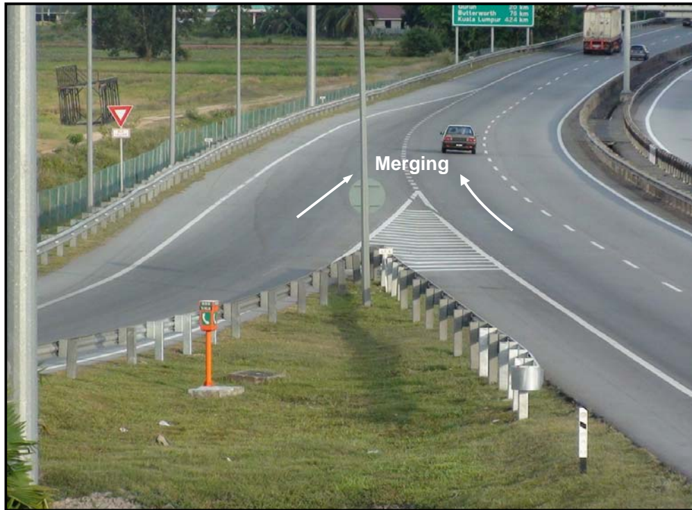
Figure 6.1: Typical on-ramp junction in Malaysia
