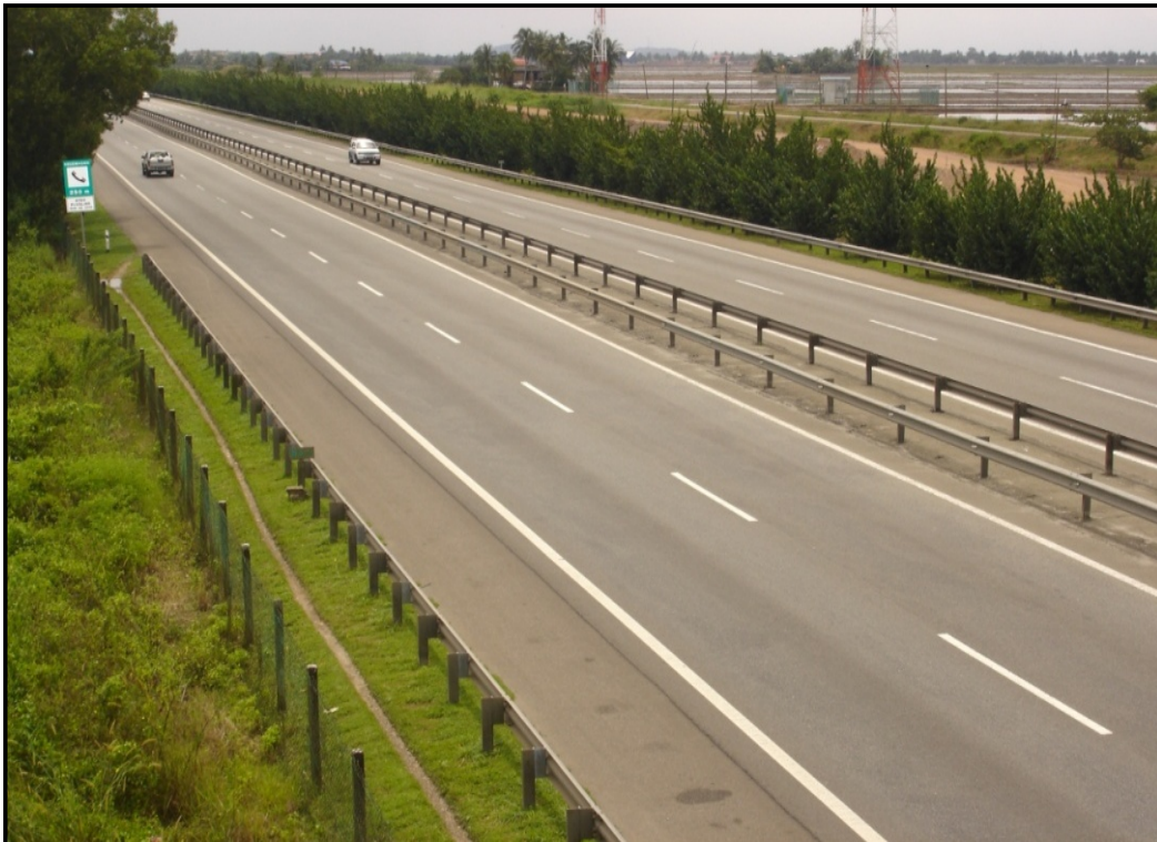
Figure 5.1: Typical four-lane basic segment expressways in Malaysia
