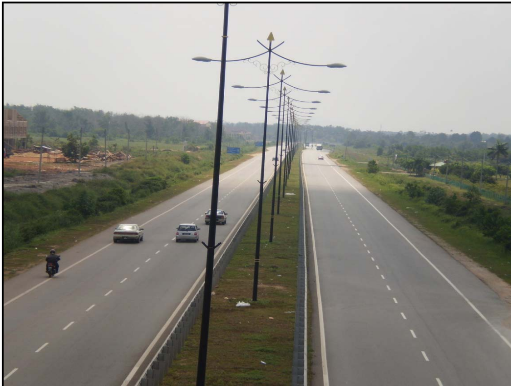
Figure 4.1: Example of a divided multilane highway in Malaysia
