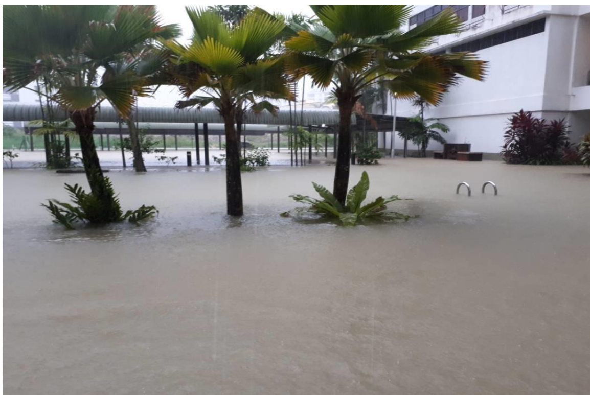
Figure 3.26: Pangsapuri Saujana (Flood Event 4 th - 5 th November 2017)
