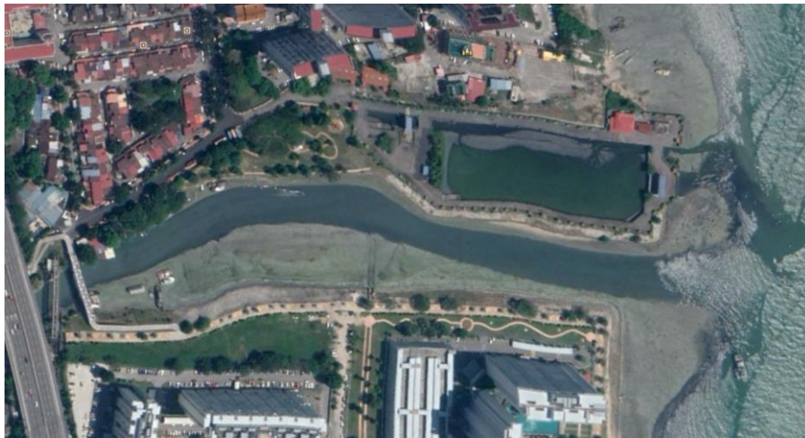
Figure 2.21: S18 Pond and Pumping Station
