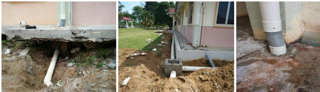
Fig. 10. The installation of the flexible joint
