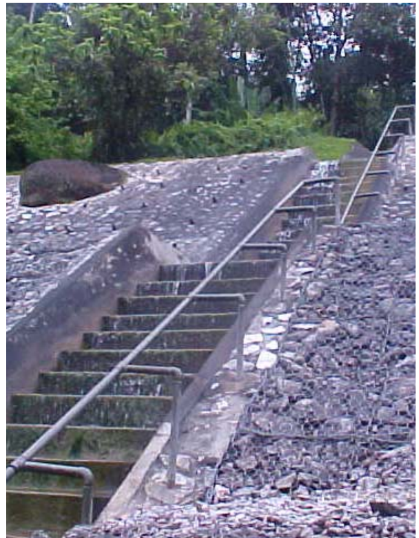
(d) Combined Stepped Channel and Stairway
