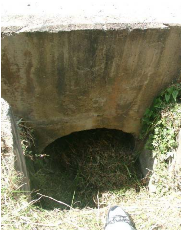
(c) Culvert at Toe of Slope
