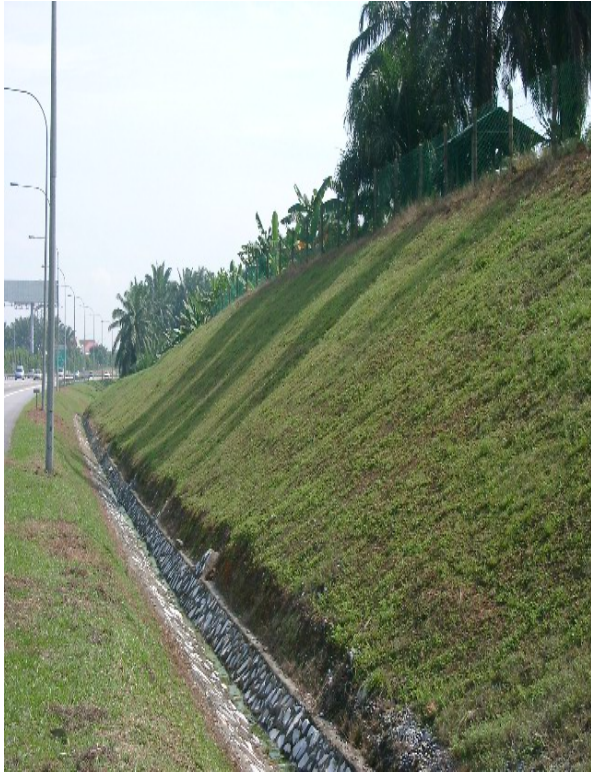
(a) V-drain along Toe of Slope
