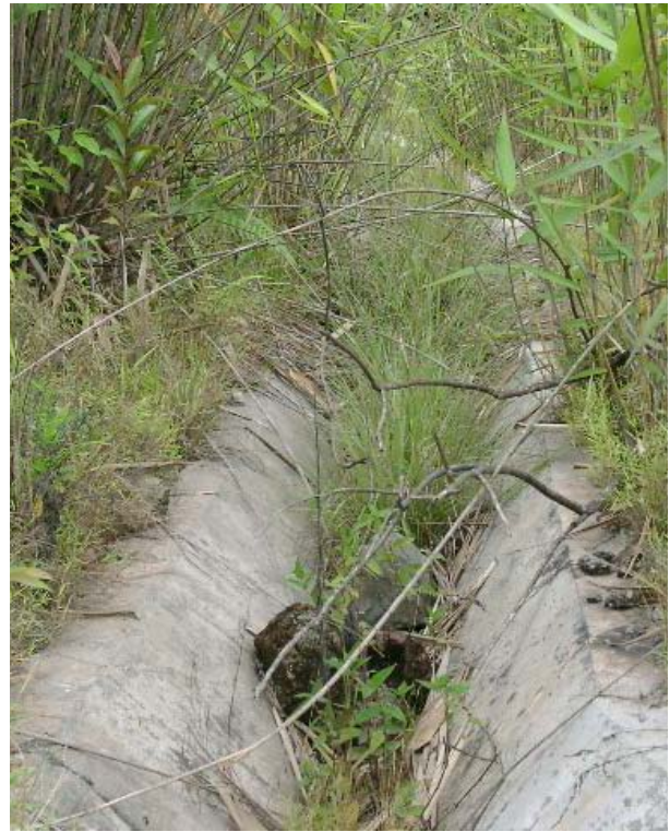
(b) V-drain along Berm of Slope
