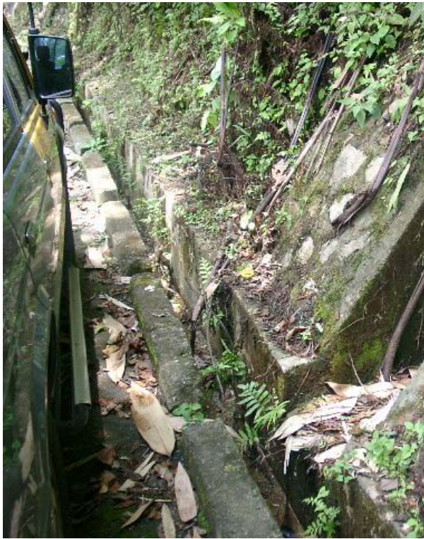
(a) U-drain at Toe of Slope
