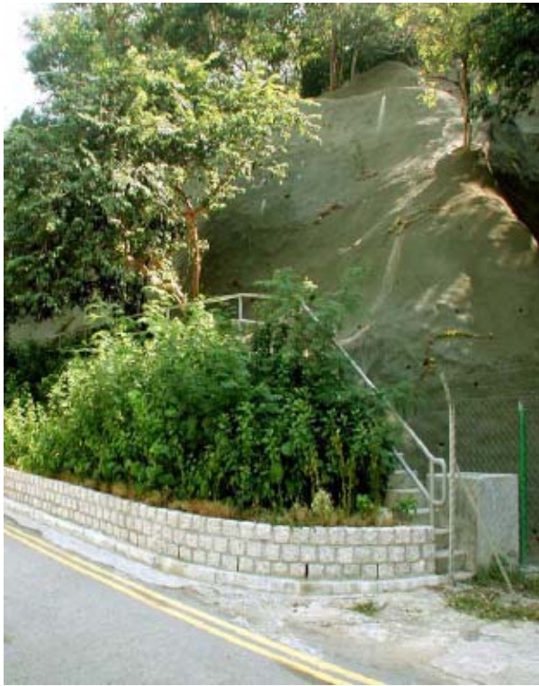
(a) Concealed Access to Stairway
